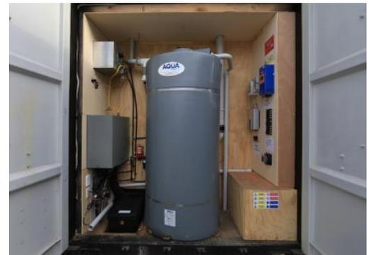
*Utilities cupboard in end of container. Contains 1000L water tank, pump and accumulator tank, first flush diverter, grey water filter system and pump, gas bottles, water heater, batteries, solar controller, inverter and electrical components.*
